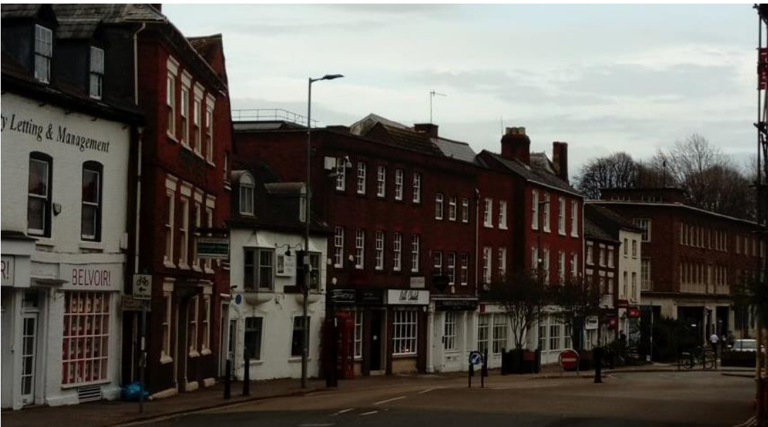
Photograph 14 view of existing museum roof from King Street
