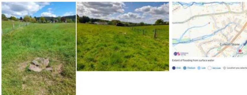
Figure 4: Site photos of culverted land drain indicated by an area of corrugated iron overlain with concrete, and an indication of its location with regards to the surface water flow route.
